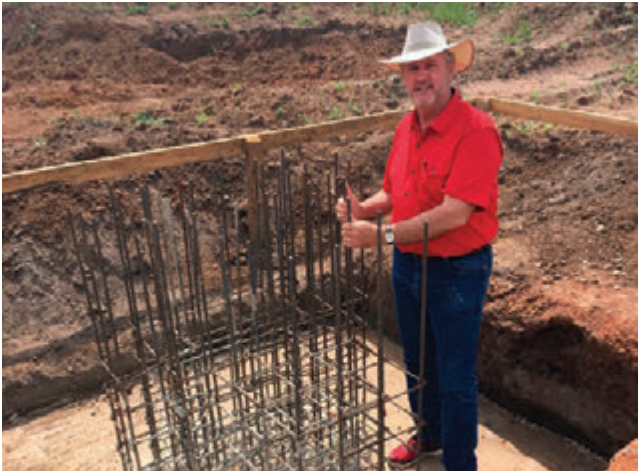
Shawn Tyler stands at the foundation of Livingstone International University as the footing is poured.
